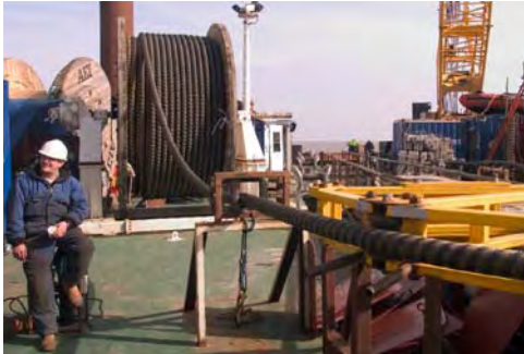
Figure 4: Cable installation from barge. Photo: Chris Laurens
