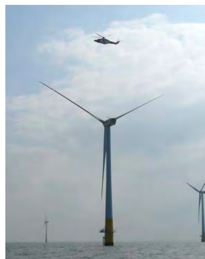
Figure 12: Vestas Offshore. Photo: Andrew Dever.
