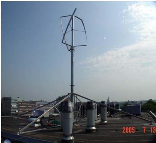
*6 m spring supported galvanized steel mast*
